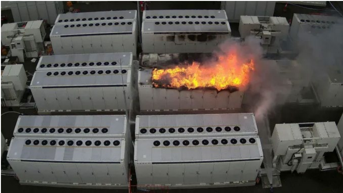
Figure 2. Thermal Runaway Fire on a Battery Pack
