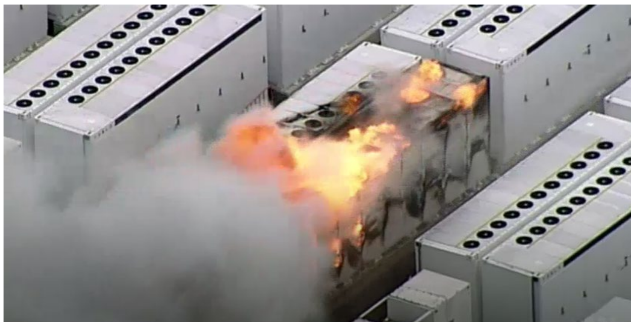
Figure 1: Photograph of Moorabool thermal runaway fire
